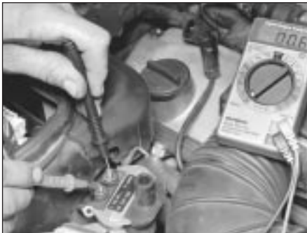
9.4c . . . using an ohmmeter, measure the resistance between the primary terminals of the coil
